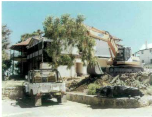
The bulldozers razed all but the original building.
