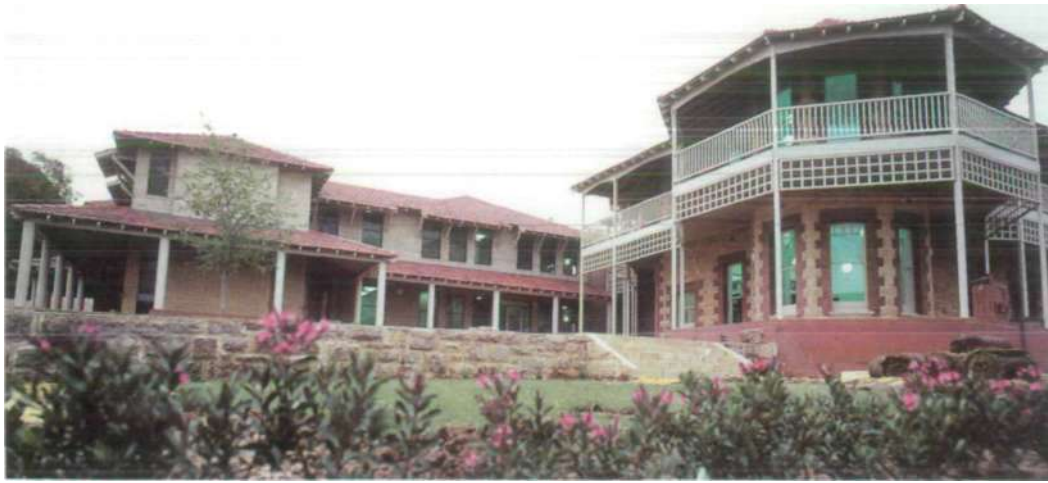
Walters House was redeveloped last year and officially opened on Speech Night 1997. The splendid original 1890s two-storey limestone residence has been retained at the heart of the precinct. Spacious and well defined living, sleeping and study areas adjoin the historic home and these are linked by a magnificent foyer.
