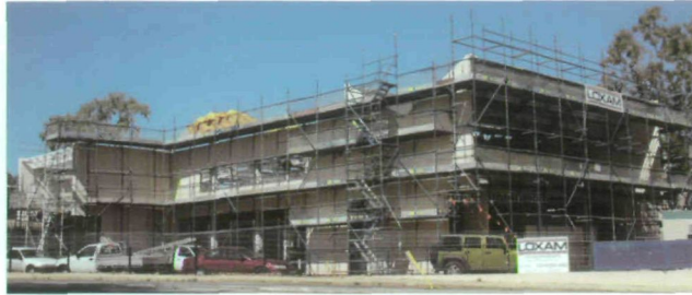
Design, Technology and Visual Arts Building takes shape.
