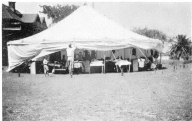
"THE TENT" which was the home of the Junior Boarders for two months while Romsey was being altered.
