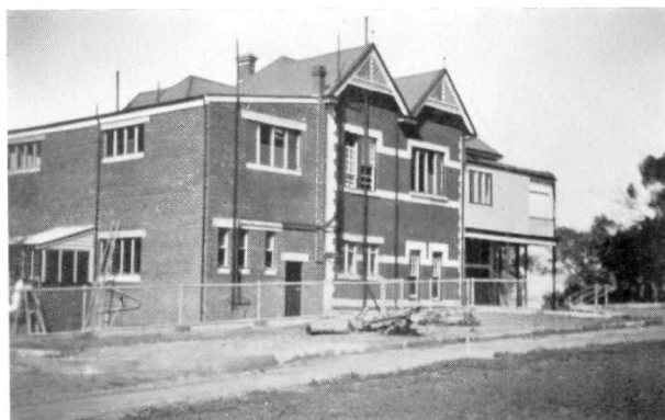
Romsey House, showing the new section at the back which was completed in August.
