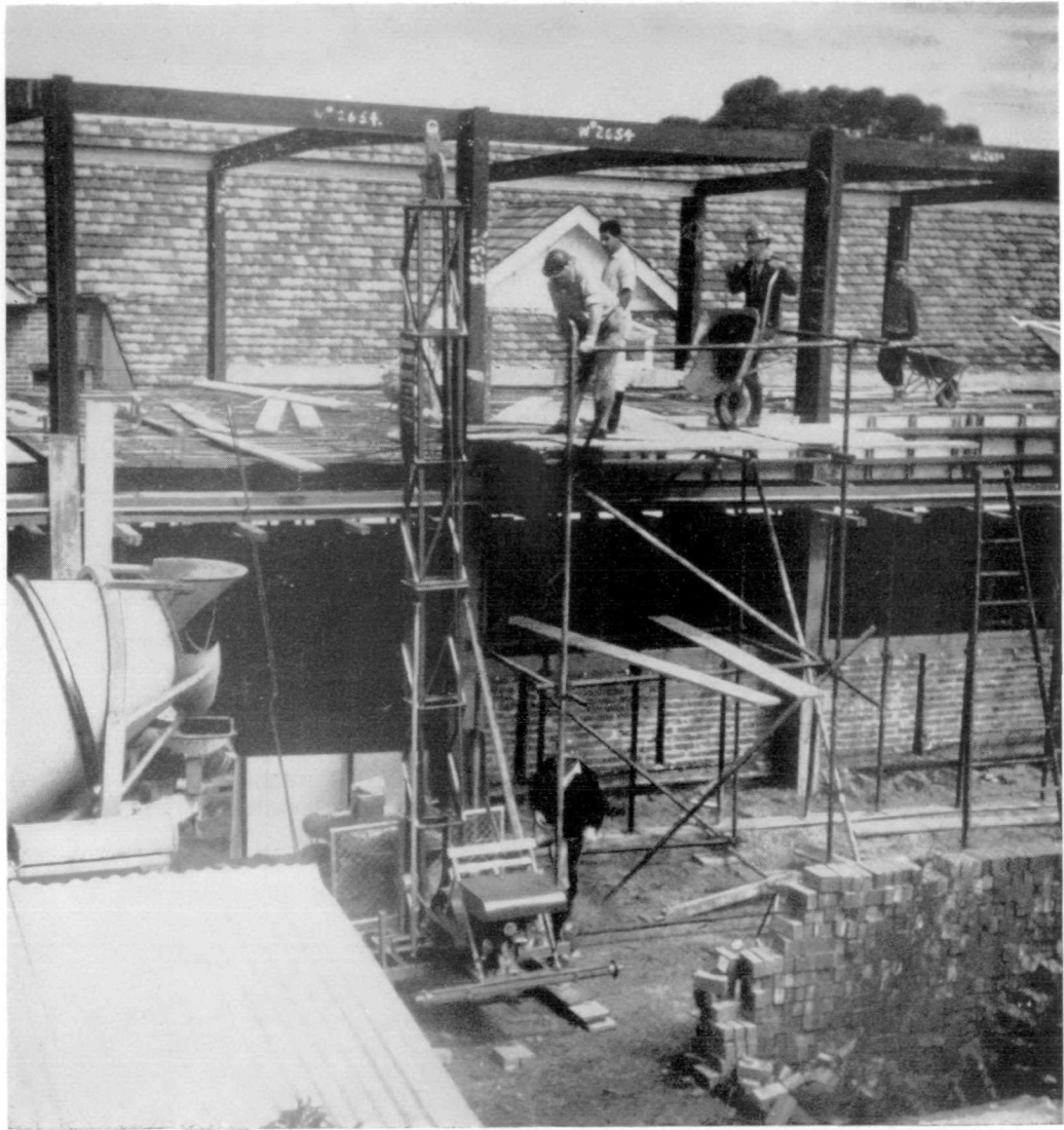
The new Science Block in the process of erection.
